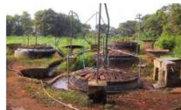
Gambar 4 Proses Penimbunan Digester ,Bak Control,Lubang Inlet,Lubang Outlet
