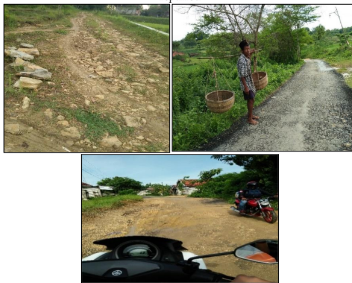
Figure 1 Situation and condition of banjar village roads, after being repaired, 1 month after being repaired
